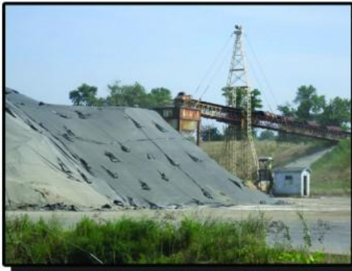
Ground Pile w/ Tie downs and sand bags
